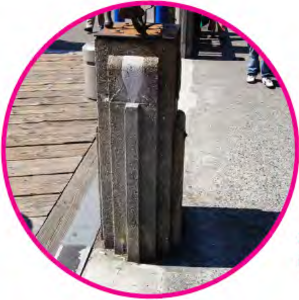
Side joint slides into railing base joint
