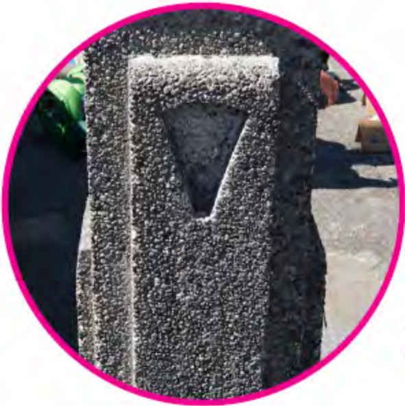
Unique joint design for top rail connection
